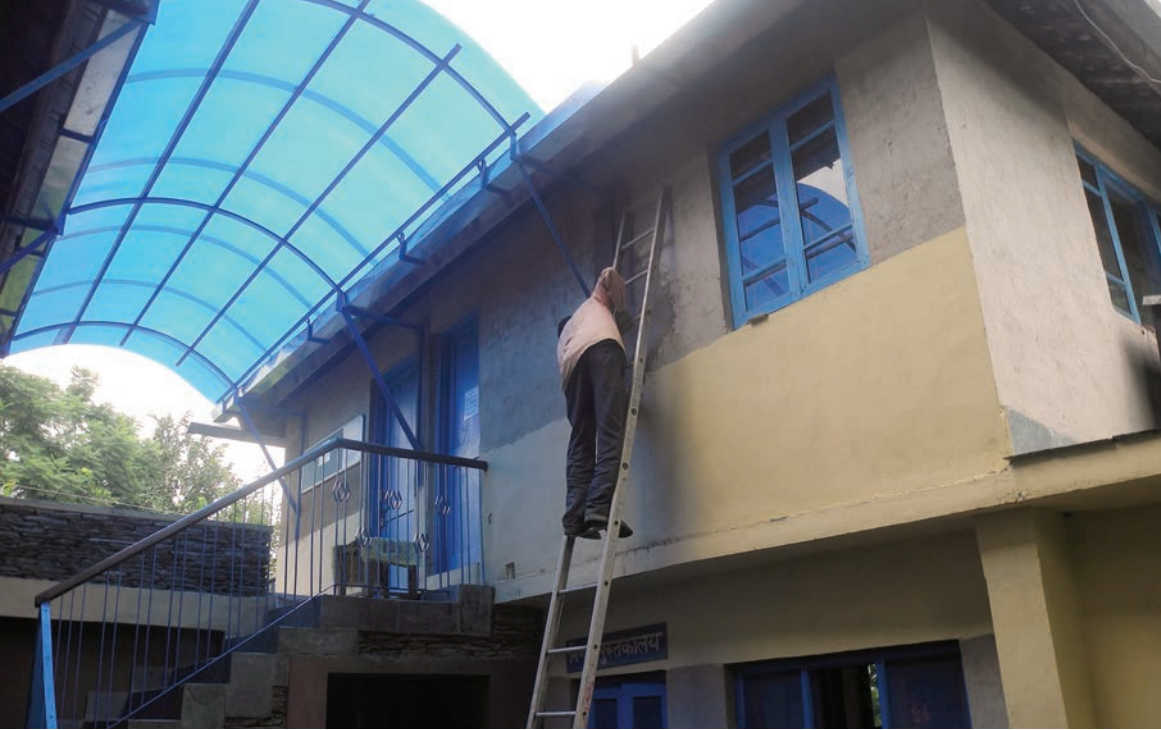
The new roof over the stairs and terraces at Nishtha community Centre.
